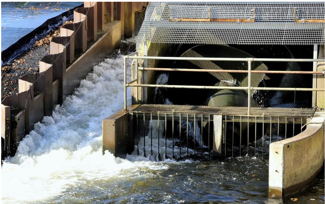
Archimedes Screw generating power at Philiphaugh, Selkirk
